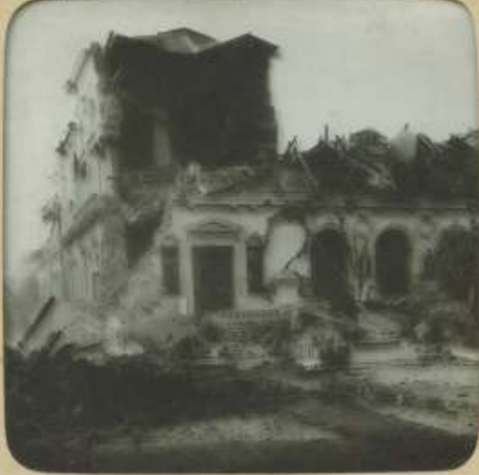
Victoria Hotel - Valparaiso earthquake -
